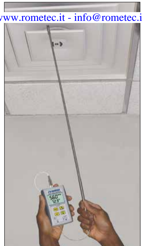
Measuring air flow from an air conditioning duct.
